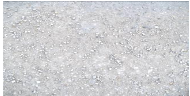
Fig. 2(a): Smooth asphalt road surface
