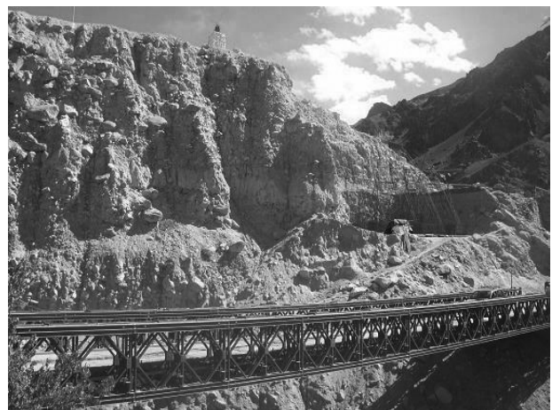
Bailey bridge in Ladhak
