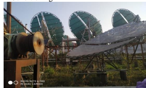
Fig.6 Solar air conditioning
