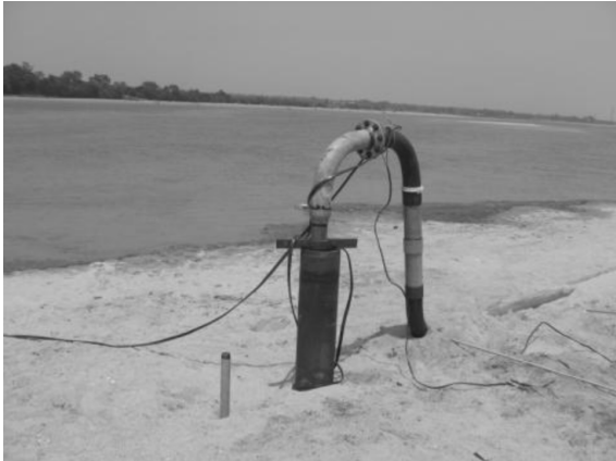
Fig. 7 Image pumping well
