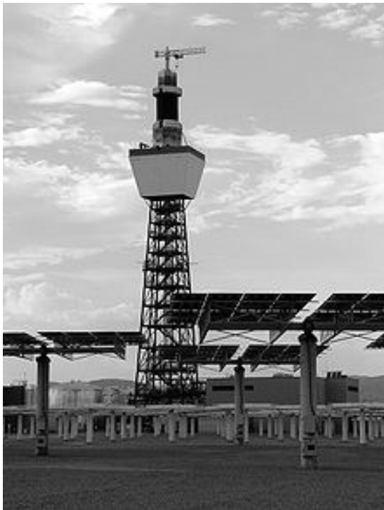
Fig.2 Solar tower with flat type tracking mirrors
