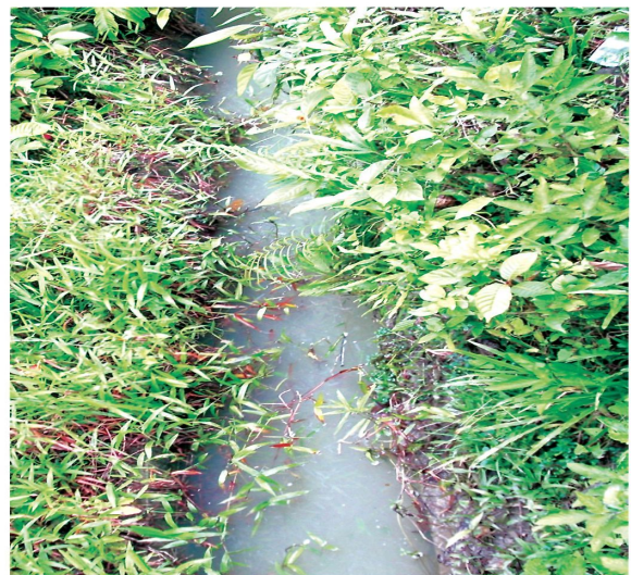
Rain water drainage on Ring road
