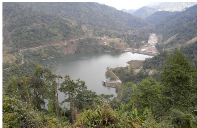
Figure 4. Ranganadi dam and downstream.
