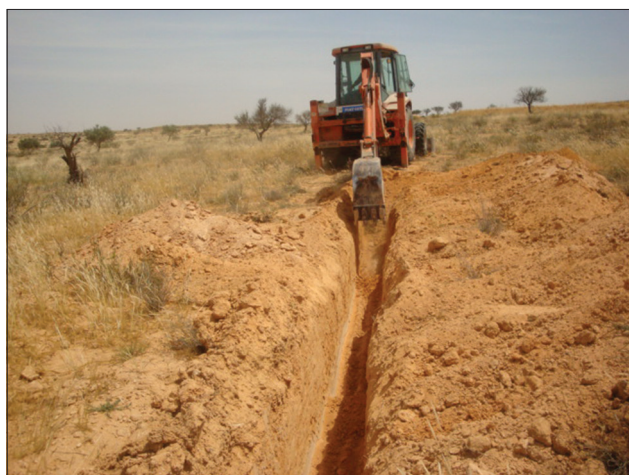
Figure-6: Preparation of AGB trench.
