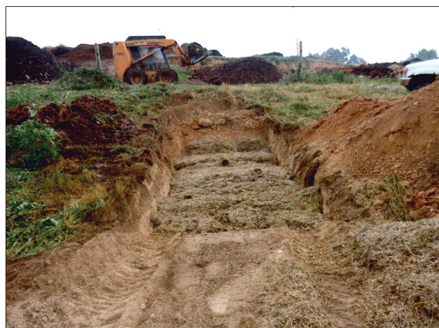
Figure-2: AGB trench ready for carcasses.
