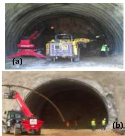
Figure 3. Tunnel excavation (a), lining concrete (b)
