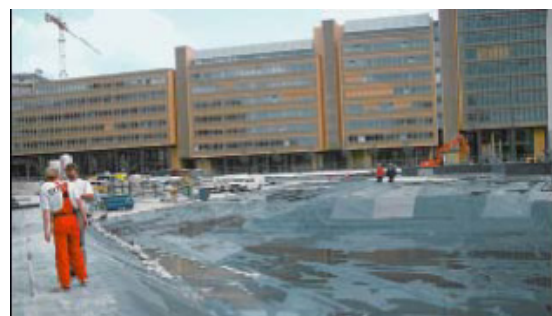
Fig.7. Constructed on top of a traffic tunnel, the biotope is lined with a geomembrane ( www.scribd.com/doc/50364355/Living-Systems )
