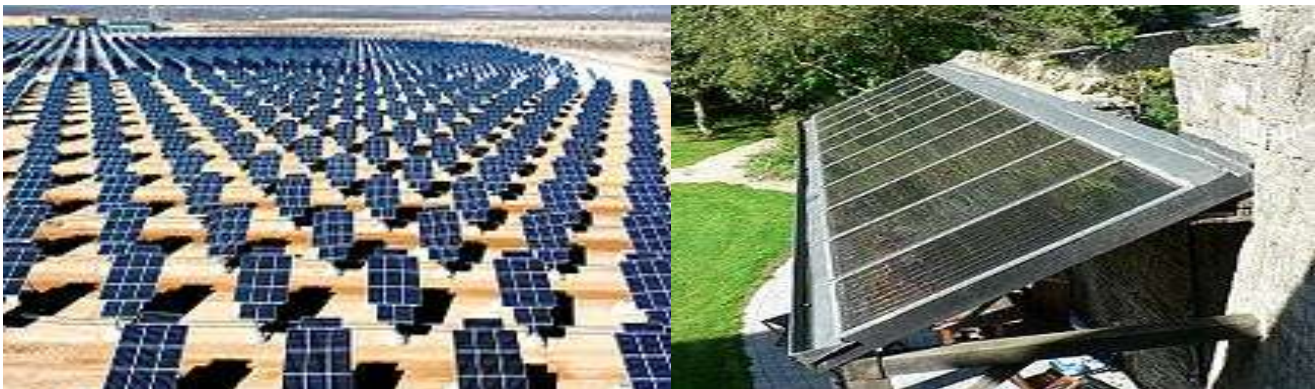
Figure 1. Photograph of PV Solar Power Plant (on Left) & Solar Water Heating Plant (Right)
