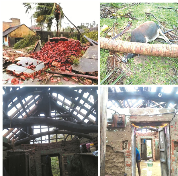
Fig. 4 — Extent of damages documented off the Nagapattinam coast, Tamil Nadu
