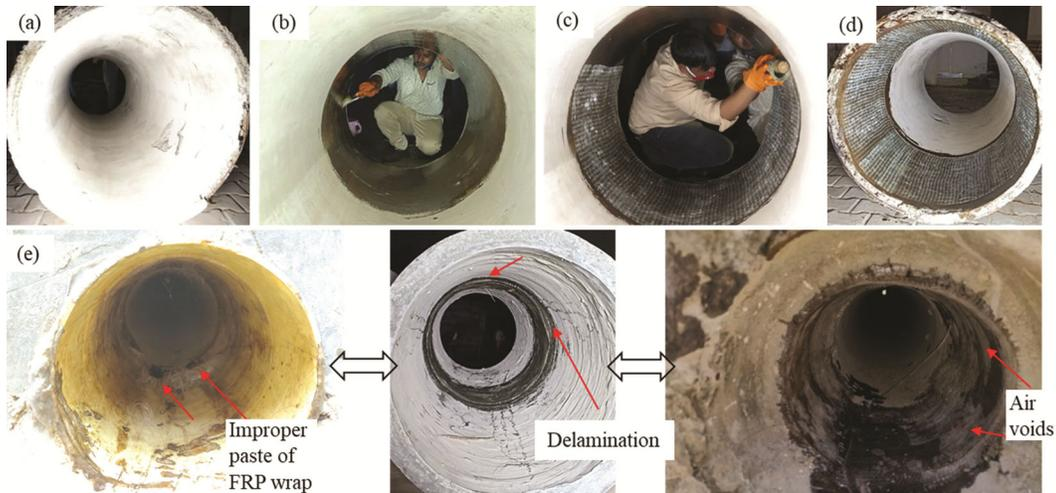
Fig. 3 — Manual FRP retrofitting strategies of sewer pipes
