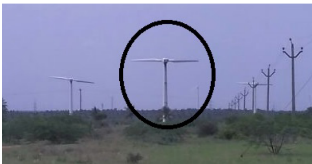
Figure 2. Awo Bladed Turbines at Dharapuram site.
