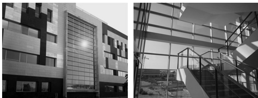
Figure 4. Exterior and interior views of the monitored active water-flow curtain wall in Cuenca, Spain.
