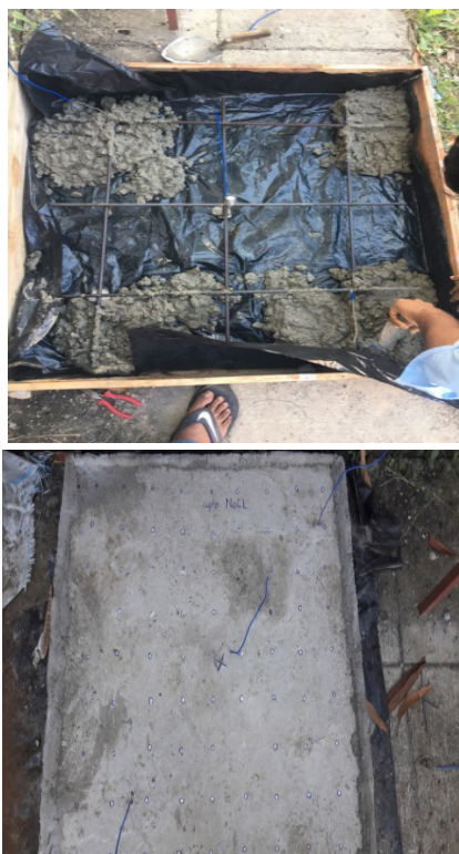
Figure 1. Reinforcement assembly with anode, slab without NaCl.
