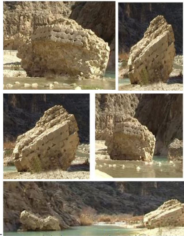
Fig. 10 . The remained parts of a bridge belonging to Sassanid period at Firooz Abad
