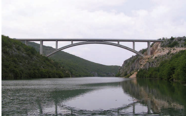
Figure 1. Aerial view of bridge.
