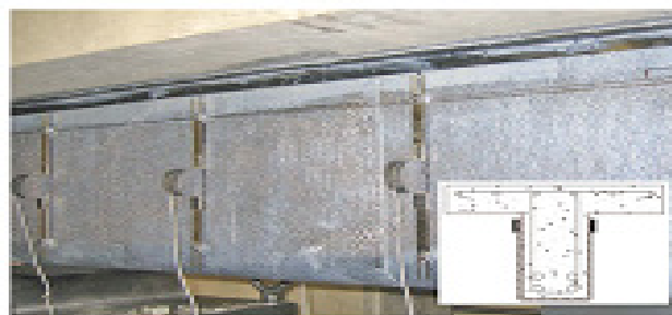
Figure 10. Alam: Elevation with surface-bonded CFRP laminate end-anchorage system 31 .
