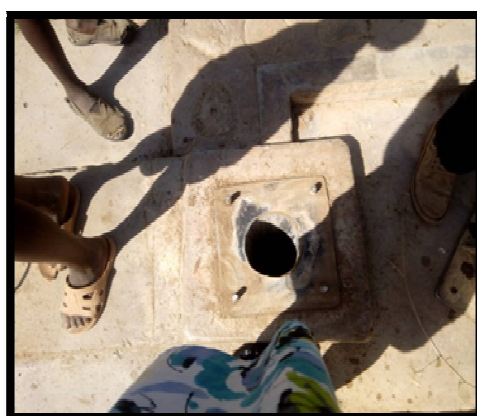
Figure 4: Hand Pump Vent under Repair
