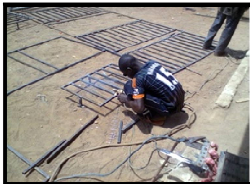
Figure 27: A Metal Design and Fabricator Welding a Window Frame
