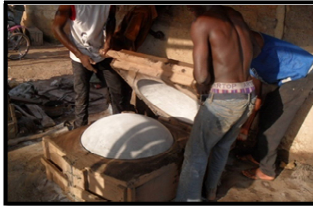
Figure 15: Fixing of the Bottom Mould of the Metal Pot
