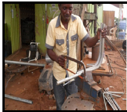
Figure 5: Cutting Taking Place
