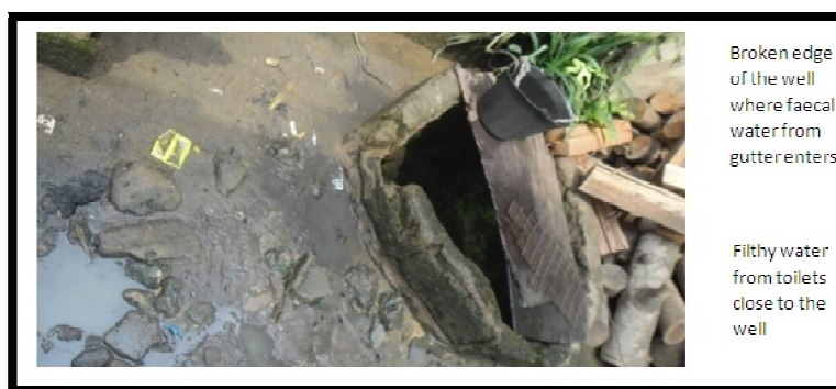
Figure 3: Broken Well Near Disposed Wastes Containing Excrements at Bepanda (Source: Kah Evans)
