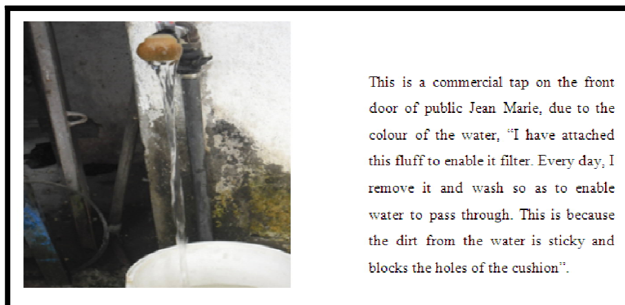
Figure 7: Adapted Local Cushion Filter of Tap Water in Nylon, (Source: Kah, 19th September 2012)
